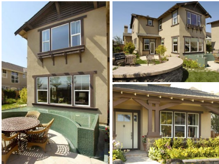
Complex window and door compositions with wood detailing
