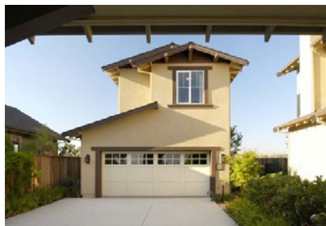
Garage door treatments echo the Craftsman style through use of wood framing, windows, and lighting fixtures
