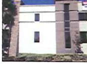
10. LOOKING SOUTHEAST- WEST SIDE OF BUILDING FACING VAN BUREN
