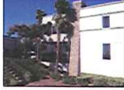
9. LOOKING EAST- WEST SIDE OF BUILDING FACING VAN BUREN
