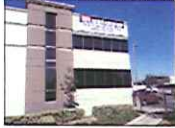
11. LOOKING NORTHEAST AT EDGE OF SIDEWALK ON VAN BUREN
