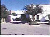
6. FACING SOUTH- FRONT SIDE OF BUILDING
