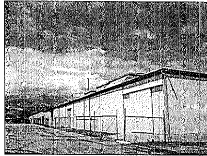
BUILDING B & C REAR - 1
