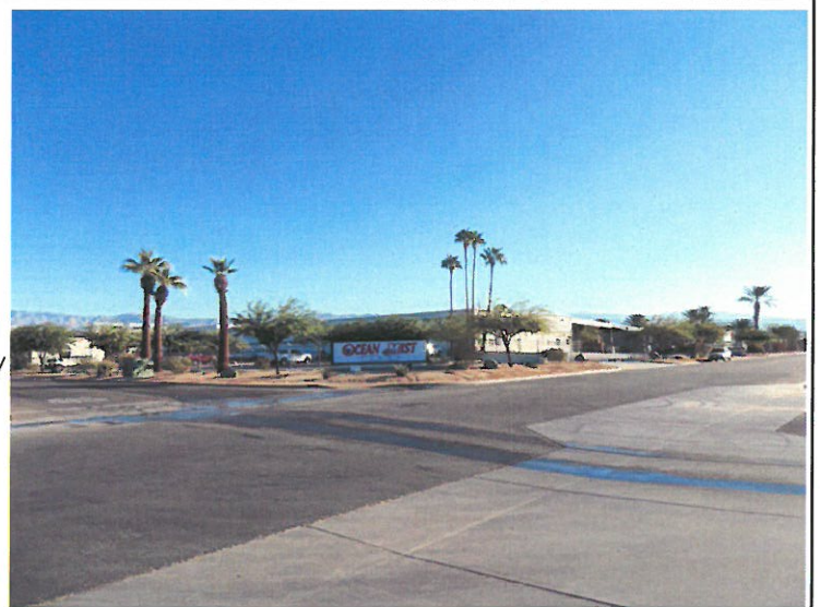
Photo 4: View of Ocean Mist facility from north west corner of Industrial and Enterprise Way facing north east
