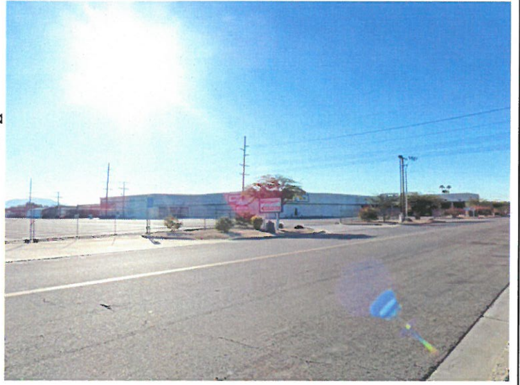
Photo 8: View of the shipping area facing south east
