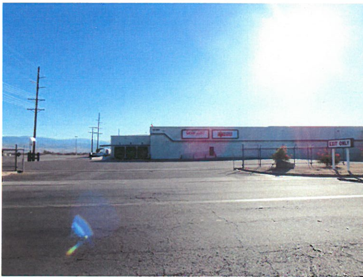
Photo 5: View of west side Ocean Mist facility facing east
