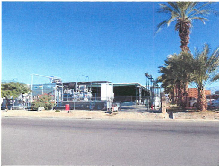
Photo 1: Facing north from the south east corner of the Ocean Mist property
