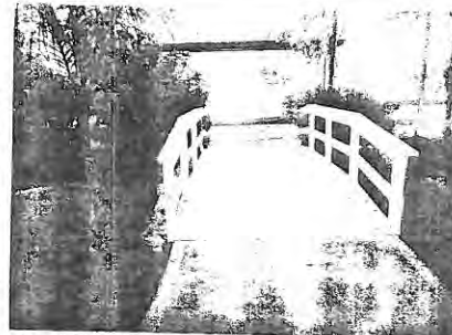
FOOT BRIDGE #1 & ENTRANCE STRUCTURE #1
