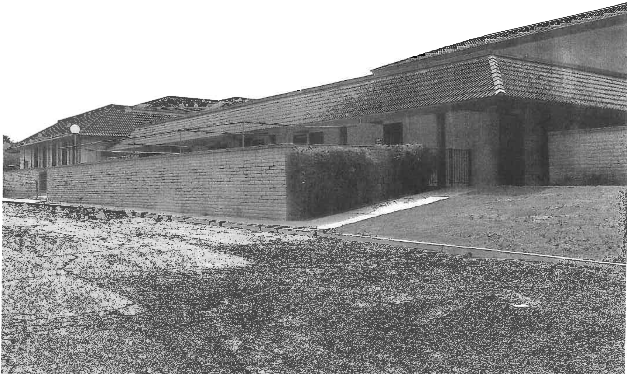
5320 VICTORIA AVE. NORTH ELEVATION
