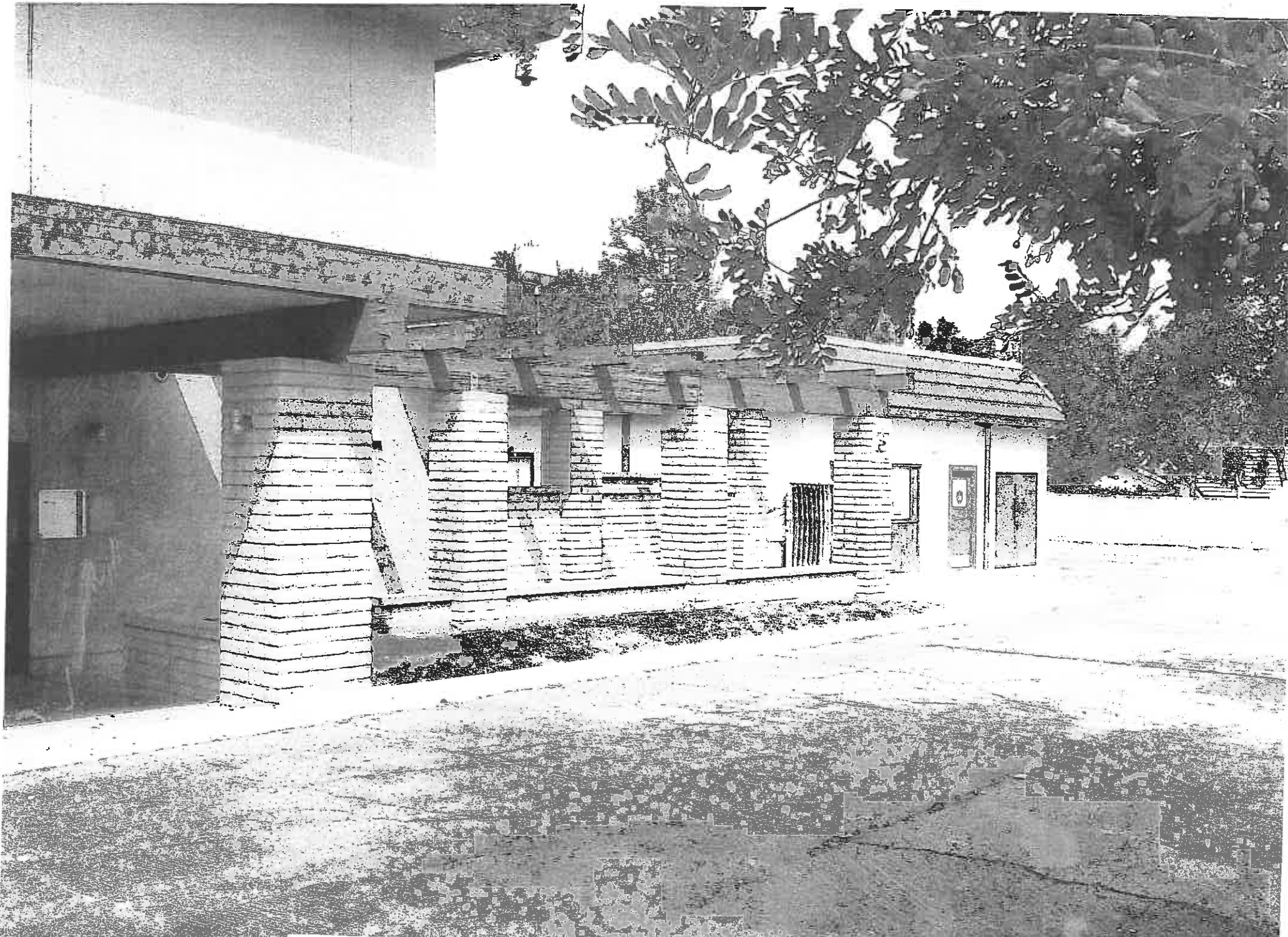
5320 VICTORIA AVE. EAST ELEVATION
