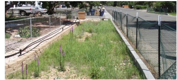
Small bioretention facilities that provide sparse vegetation may be suitable in an aviation environment.
