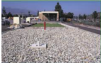
Infiltration basins with rock bottoms are less attractive to birds because they mask water and do not provide vegetation.
