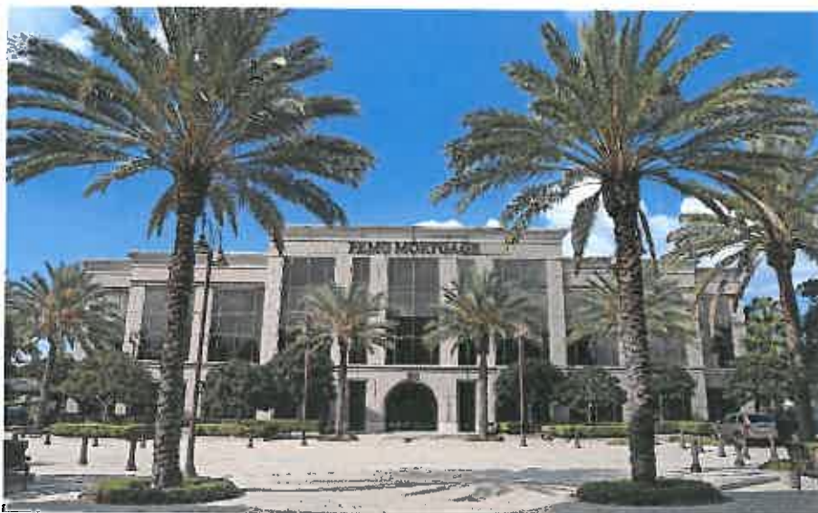
An example of multi-story office space using landscaping to frame dimension.
