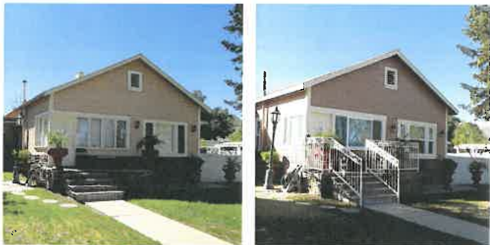
Handrails and railings improve the safety of entrances to residential units
