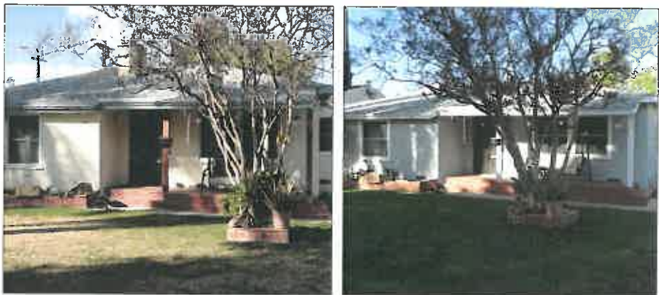
Corona's housing rehabilitation program assists homeowners in replacing roofing, painting and lead abatement, and other home improvements.
