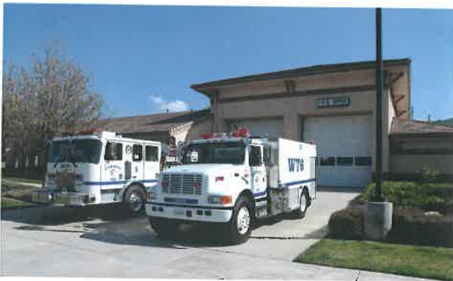
Fire Station 6, in south Corona, is one of its seven fire station locations
