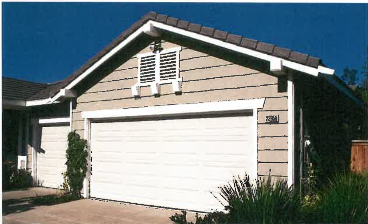
Below: Garage doors should be simple in detail and toned to compliment the building's color palette. Attention should be given to trim detail. Garage doors should be offset as shown when more than a two-car door is required.
