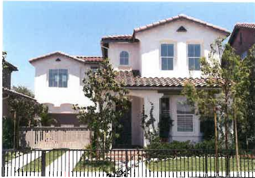
The recessed covered entry, variation in the second-floor setback and one-story roof element over the front porch provides an effective reduction in the building's mass and also provides a desirable scale along the neighborhood street. Larger visual space between adjacent homes is created by setting the garage well back from the front of the home.
