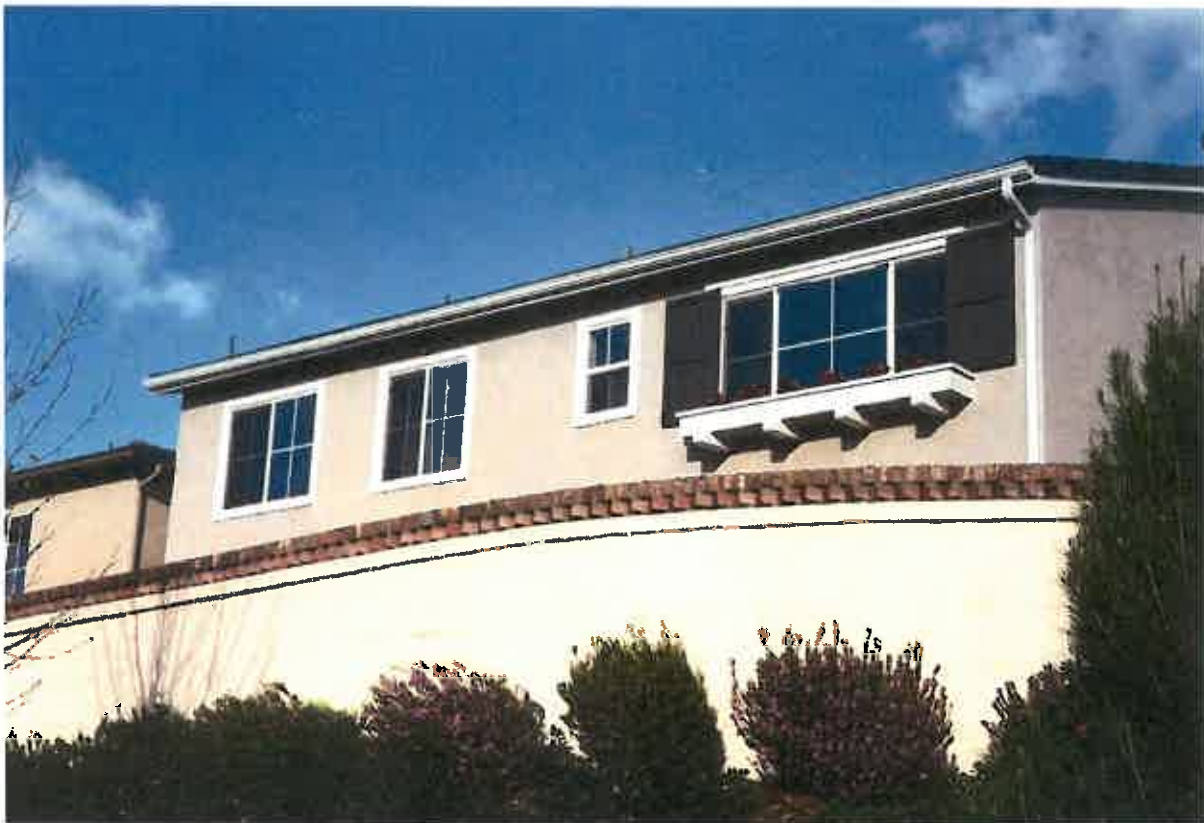
The top example shows the effective use of window trim painted in accent colors, pot shelves, architectural banding and tonal variations to enhance the overall appearance of the rear façade of the homes. The bottom example shows the effective use of accent shutters to enhance the rear window. The bracketed pot shelf is a nice addition. These types of design enhancements will be required to wrap around to the side façade when the side façade is visible from neighborhood streets, parks or open spaces.
