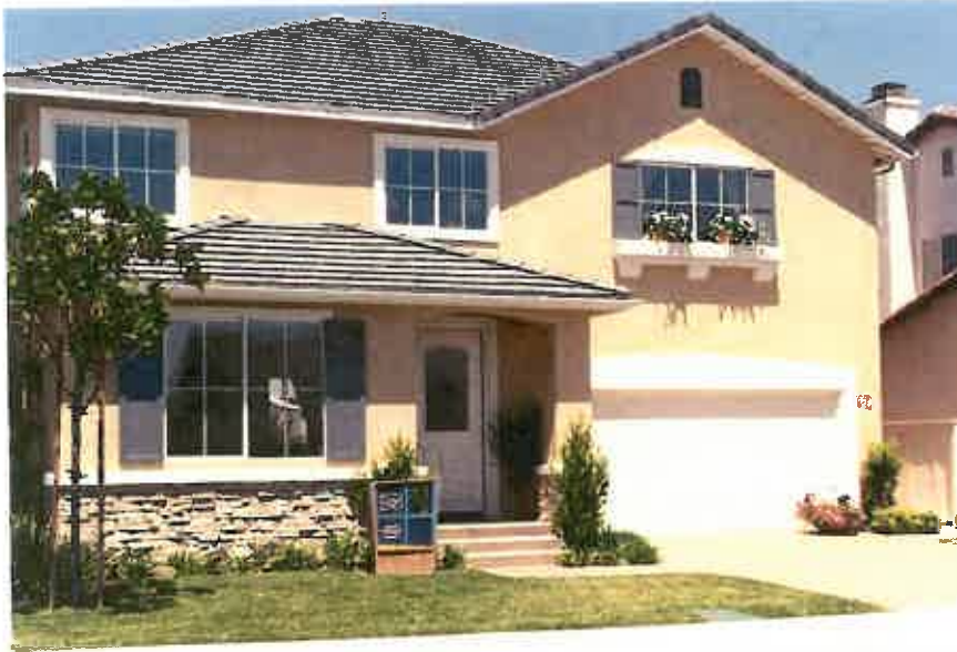
This house shows an effective use of a simple color and material palette. The primary stucco building façade, painted a light ochre color, is accented nicely with trim details and accent materials. The roof overhangs, painted white, provide a nice relief at the roof edge. The “ledger stone” that accents the base of the formal front window is complimentary to the color palette.
