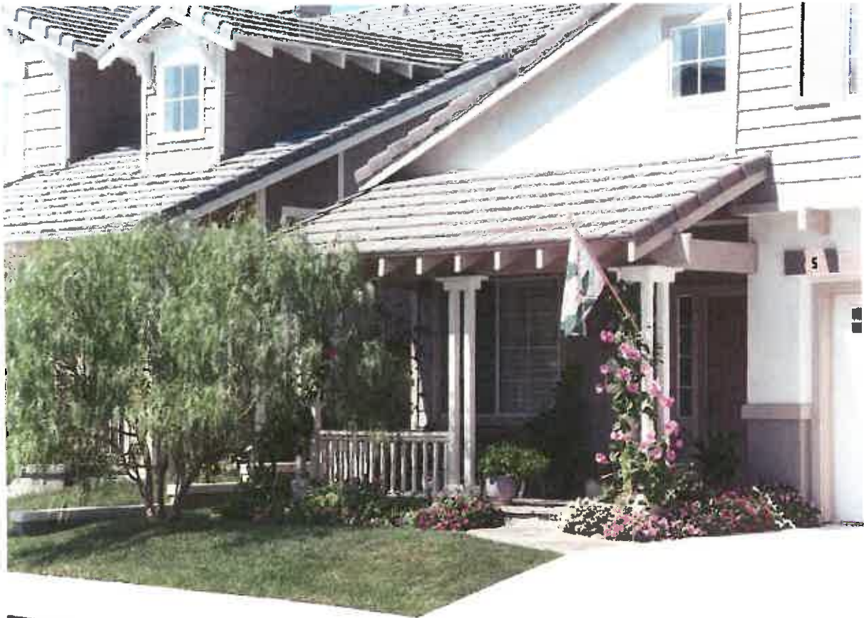
Excellent example of well proportioned, articulated and defined front porch
