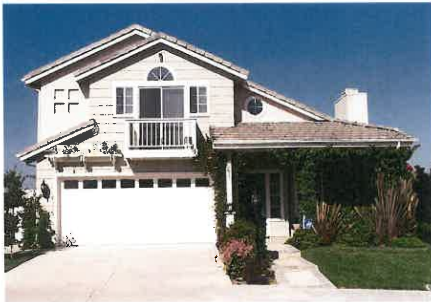
The rooflines, variation in façade setback and surface materials and the covered front porch effectively breakup the mass of this building and bring the scale of the house to the street level. The front gabled roof elements accented by the one-story porch roof are effective in combination.
