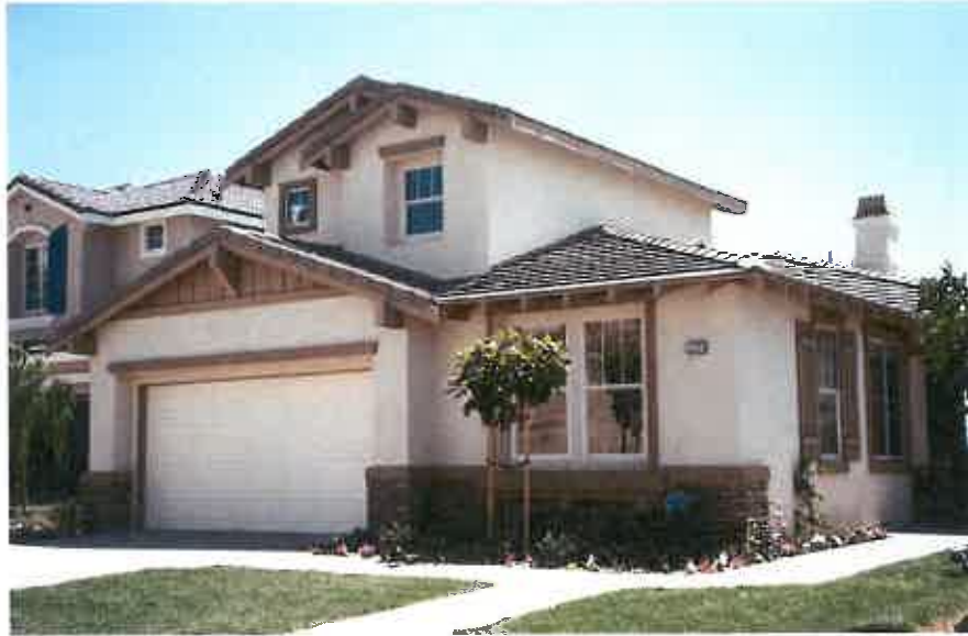
The mass and scale of this house is effectively addressed through the use of the one-story wrap around roof with front-gable and hip components, the partial second-story element with variable setbacks, and the nice use of materials, accent colors, architectural details, and window placement.
