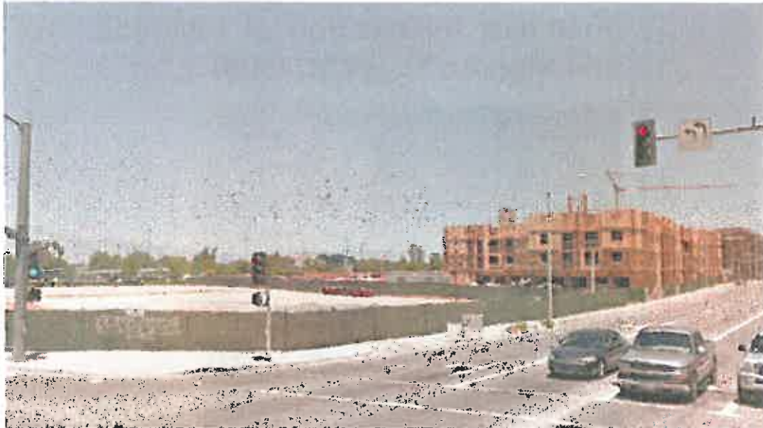
View of Site from corner of La Sierra and Indiana Avenues looking northeast
