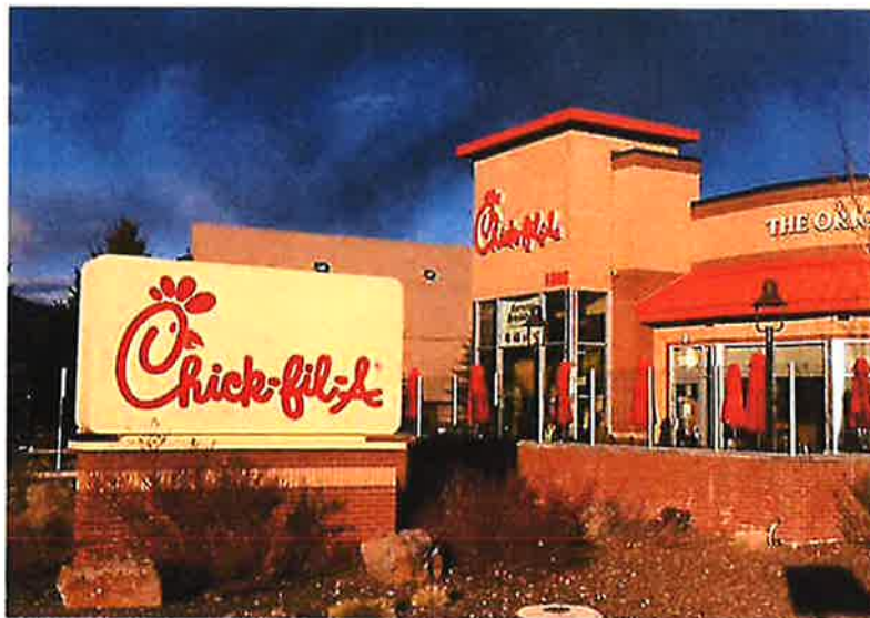
Figure 3.05.06-6, Example of a Freestanding Sign Incorporating the Architectural Details of the Main Building
