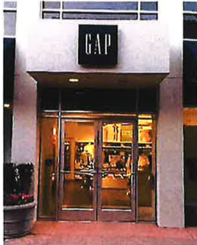
Figure 3.05.06-4, Examples of Well-placed Signs Emphasizing A Building Entrance
