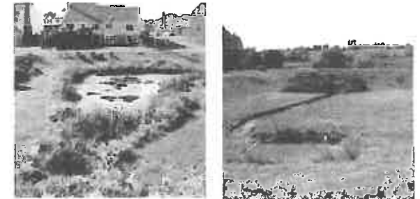
Extended detention basins are frequently used to serve both water quality management and to provide amenities. These basins hold water and would not be appropriate within an AIA because of the open water.
