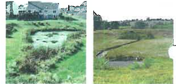
Extended detention basins are frequently used to serve both water quality management and to provide amenities. These basins hold water and would not be appropriate within an AIA because of the open water.
