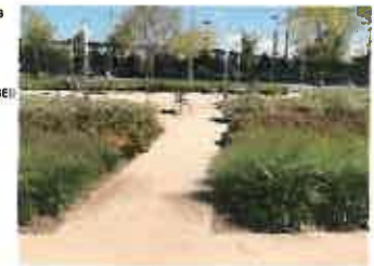
ORGANIC-LOCK STABILIZED DECOMPOSED GRANITE PAVING
