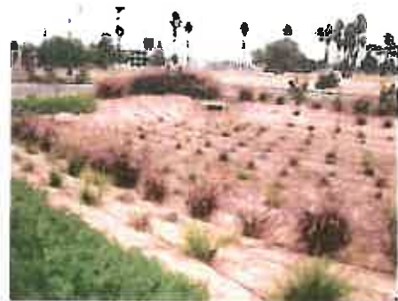
Infiltration Basin (Source: SoCal LID Manual)
