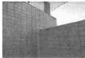
GARDEN WALL PRECISION CONCRETE BLOCK WALL COLORED
