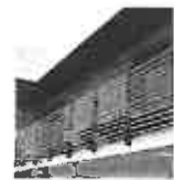
M BALCONY METAL RAILINGS
