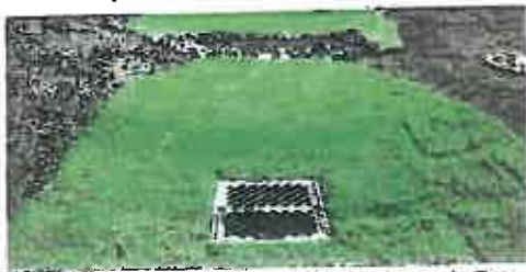
Infiltration trenches detain water for brief periods. This trench at Seattle-Tacoma Airport includes vegetation appropriate for an airport environment.
