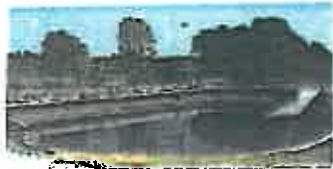
Adaptive measures such as liners, a concrete basin, and overhead wire grid can make extended detention strategies less attractive to hazardous wildlife.
