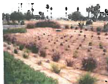
Infiltration Basin (Source: SoCal LID Manual)
