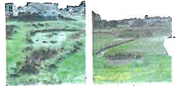
Extended detention basins are frequently used to serve both water quality management and to provide amenities. These basins hold water and would not be appropriate within an AIA because of the open water.
