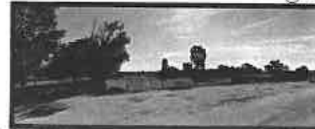
10 GARAGE ON RIVAUD RD. WITH PROPERTY BEYOND - Looking South
