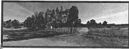
13 GARAGE ON RIVAUD - Looking Southeast
