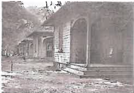
Railroad worker cottages circa 1907. Courtesy of CVWD.
