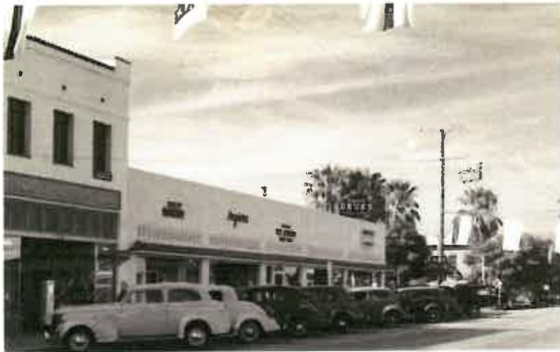
Original On-Street Parking Configuration in the Downtown
