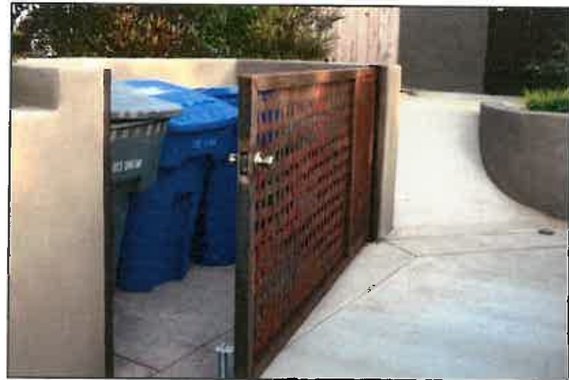
Locate refuse out of view from the public
