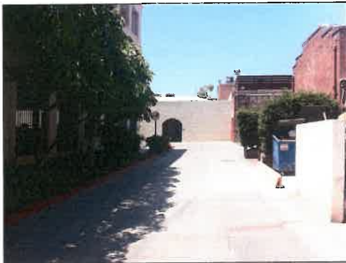
Improve rear facades of buildings
