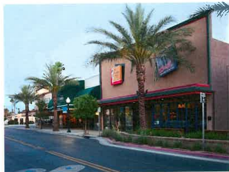
Public Improvements and Facade Rehab - Miles Avenue.
