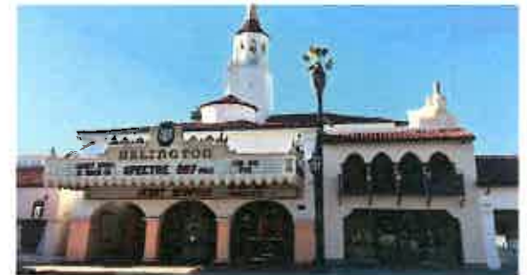
A movie theater next to retail buildings.
