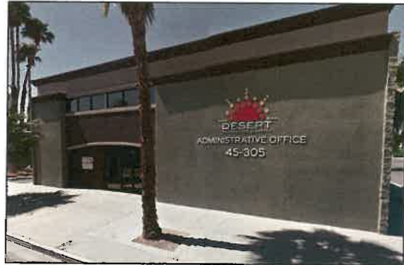
Wall signs should not project from the surface more than six inches
