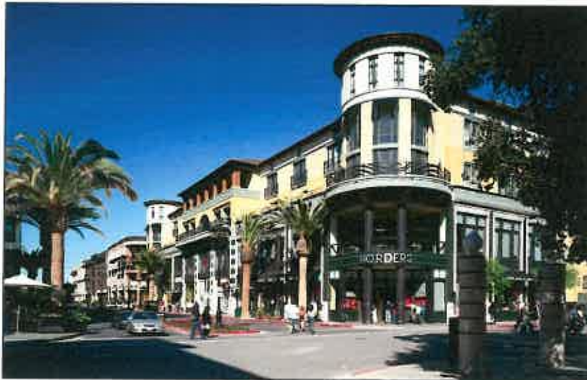
Building facades should be detailed to create visual interest
