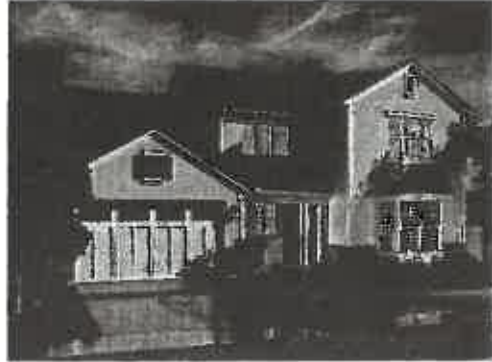
Roof design consistent with architectural style of the building
