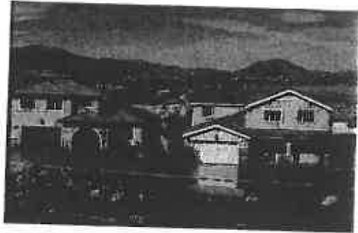
Variety in texture and color on building elevations
