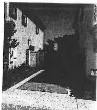
Guest parking space between buildings
