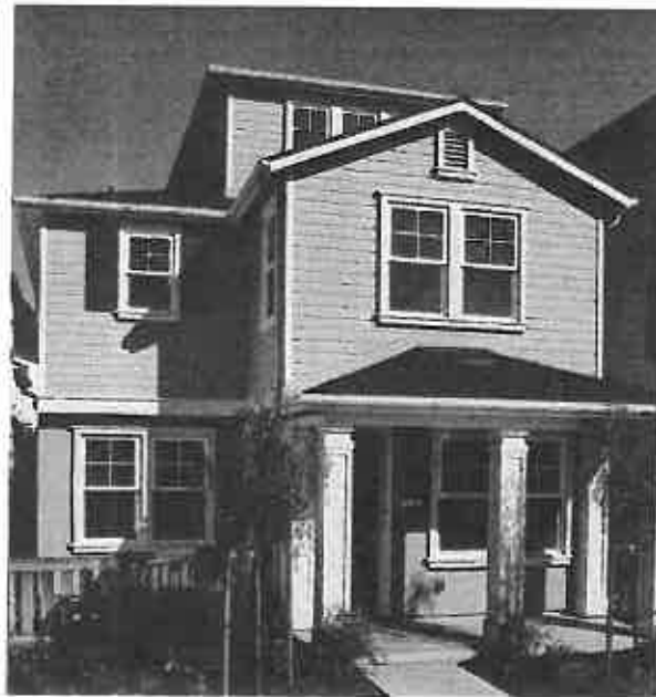
Porch, shutters and trim
