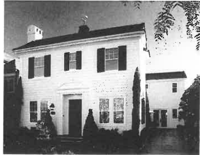
Pedimented entry shutters and window details
