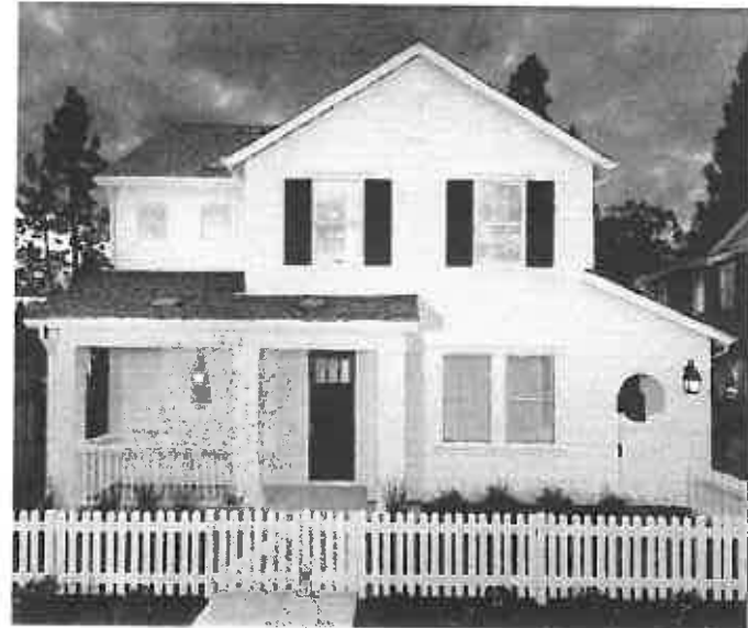
Entry porch, siding and shutters
