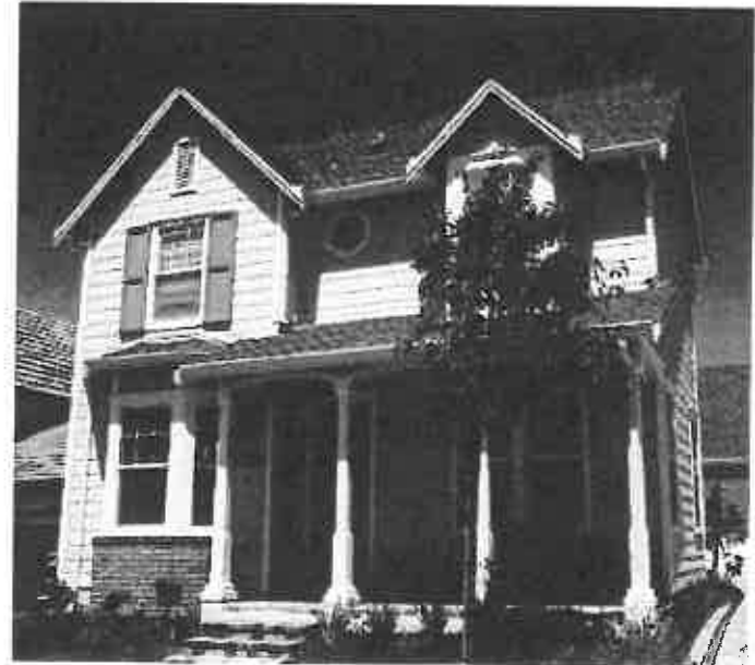
Porch, posts, materials and roof form
