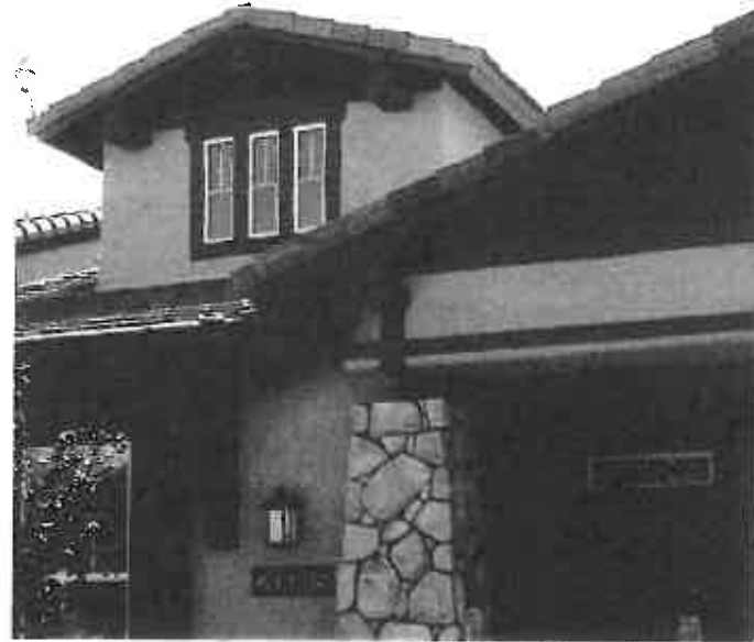
Exposed rafter tails and materials
